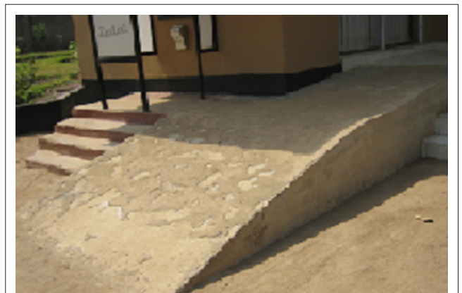
FIGURE 6: Steep ramp without rails leading to an automated teller machine at a bank.
