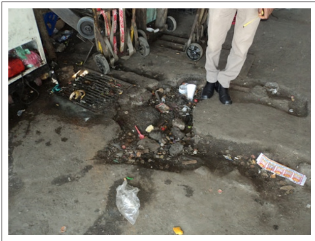
FIGURE 4: Pothole (120 mm deep and 530 mm wide).
